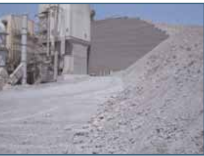
Figure 1: Crusher building (foreground), rock retaining wall (background).
